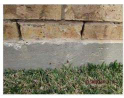
Three corners of the foundation had corner cracks. Corner cracks are diagonal, wedge shaped cracks isolated to the extreme corners of the foundation. While this is typical on concrete foundations and not considered to be a structural concern, it should be repaired, where possible to prevent further spreading. Foundation cracks require routine maintenance and may need to be caulked and/or sealed from time to time to prevent water seepage.
